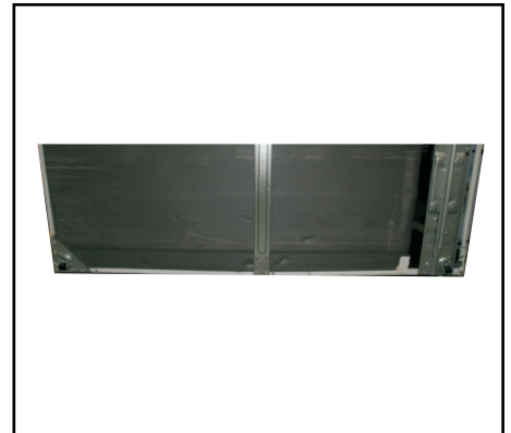
9. After completed installation.
